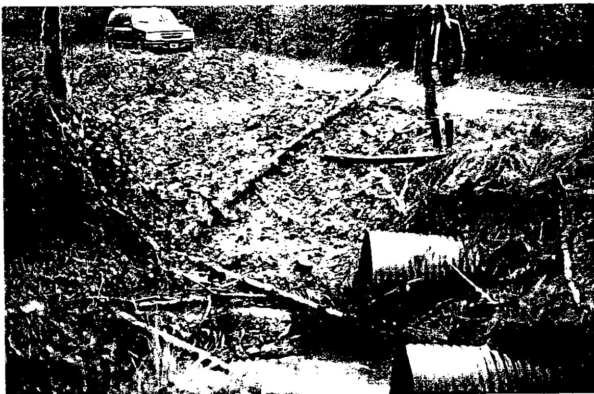
(20) Refuse pile, taken from opposite side of creek looking at quarry access road.
